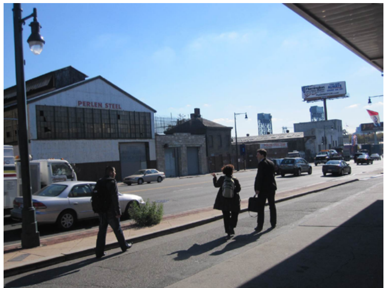
Modernizing and subdividing large industrial buildings involves high upfront costs and uncertain returns.
